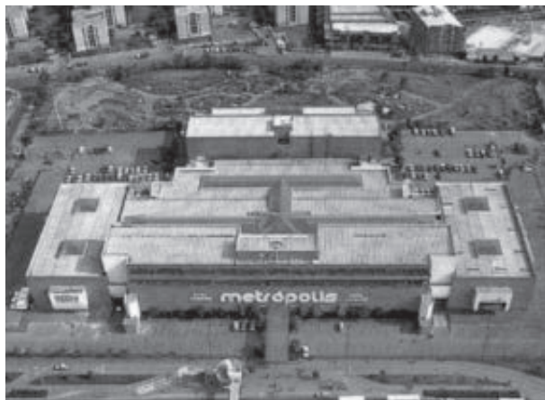
Estado original / Original condition
