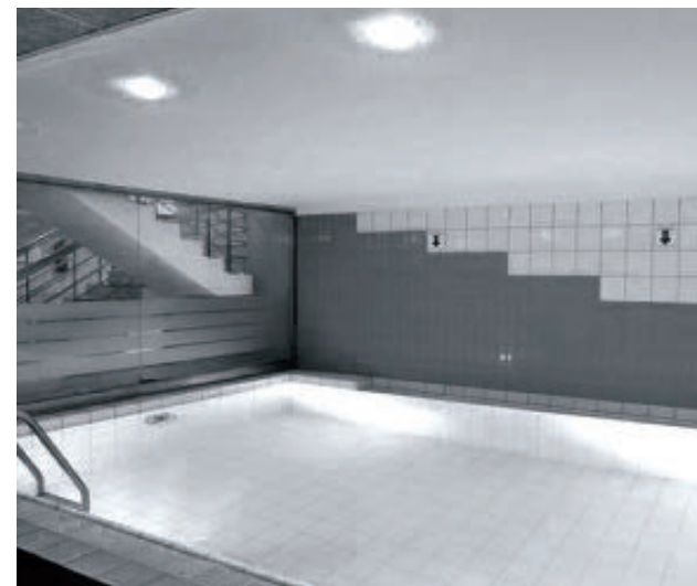
Estado original / Original condition
